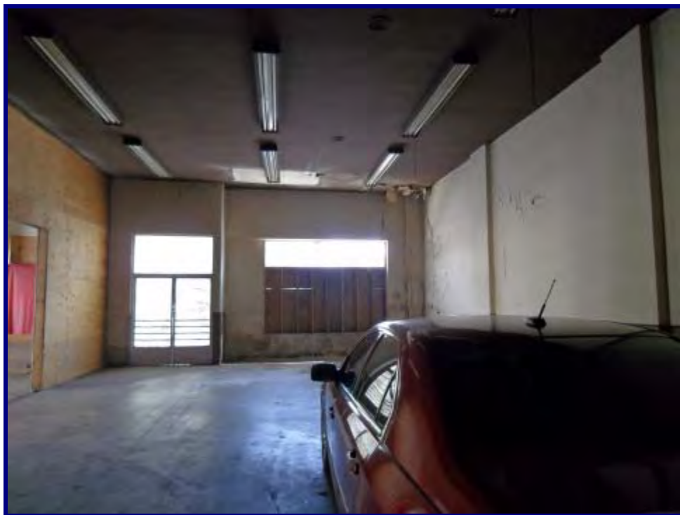
Southern lobby area
