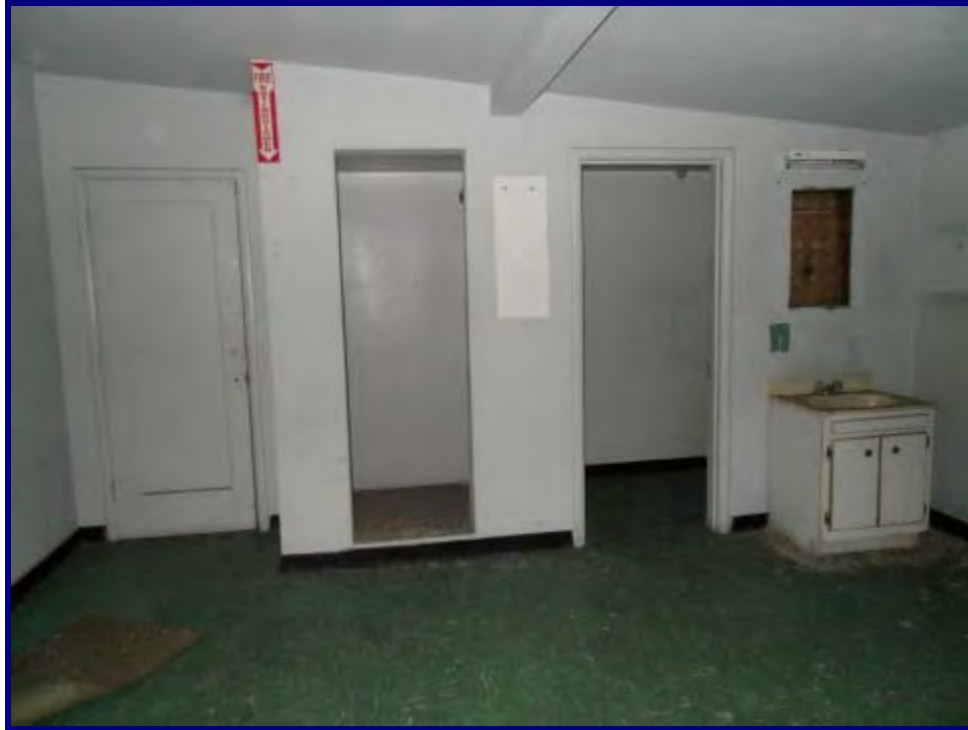
Upper level – former bus driver's room
