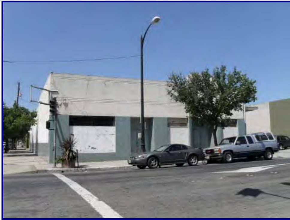
Front elevation from 10 th street.
