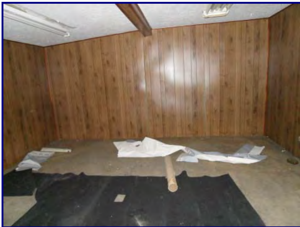
Upper level office
