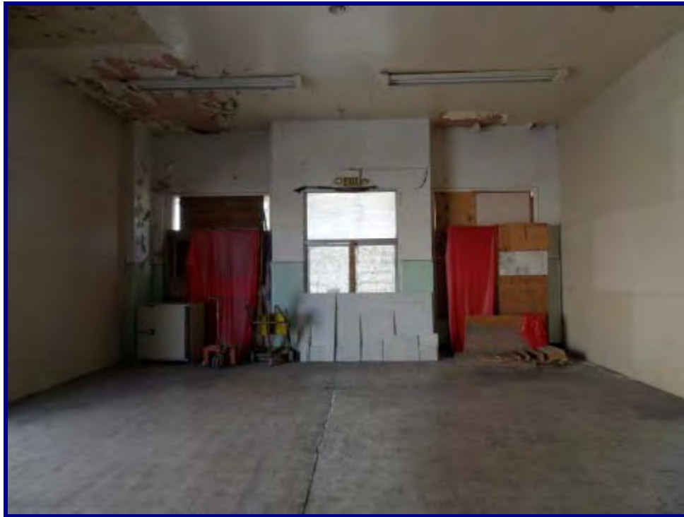
Northern lobby area (12' roll-up door to the left)
