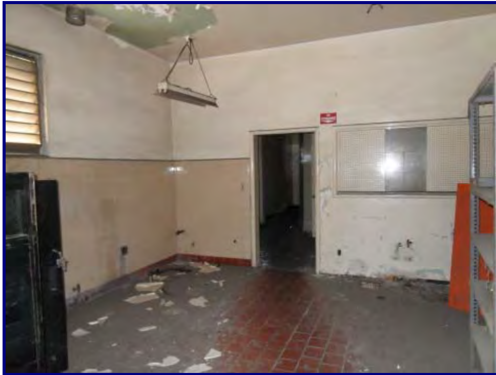
Former Kitchen area
