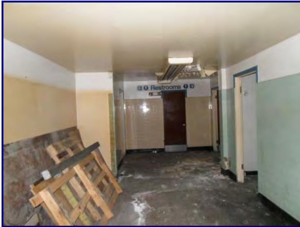
Lower level, north side hallway
