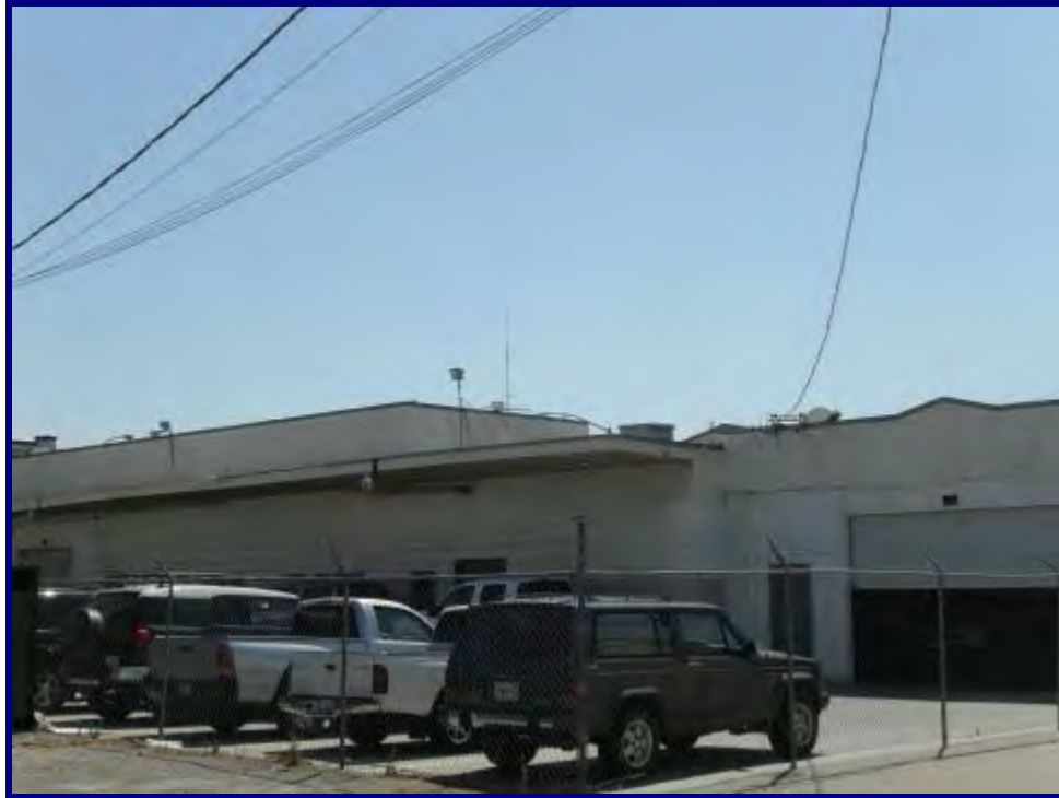
North elevation from alley.
